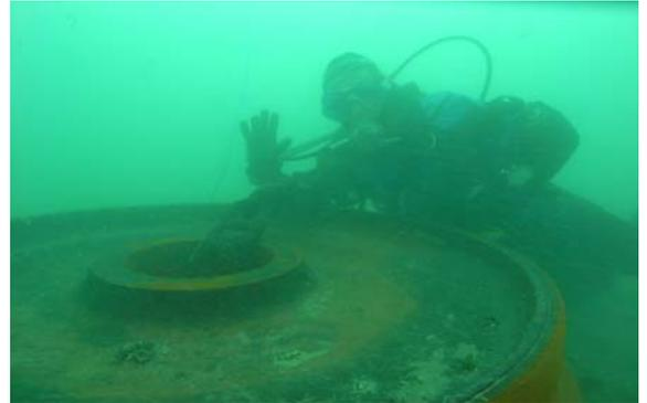
Railway wheels at the bottom of the buoy
